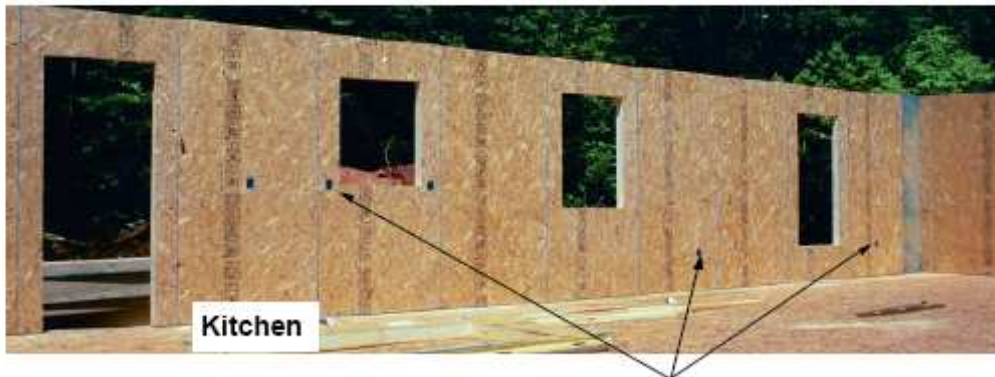
Insulation R30, door & window openings and electrical boxes ready for installation
