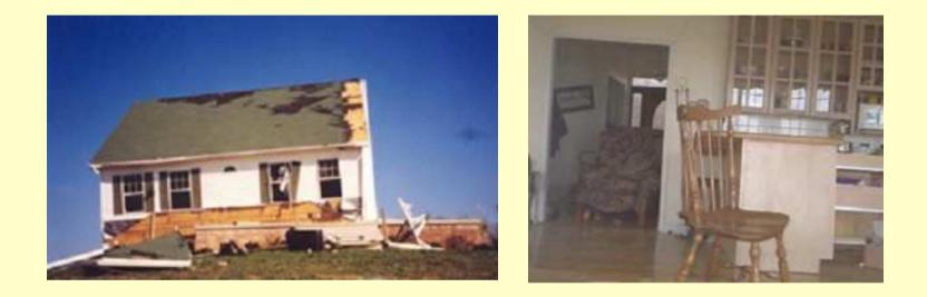
Aside from the SIP house being lifted and shifted by the tornado, the house had survived intact, with apparently very little damage.
